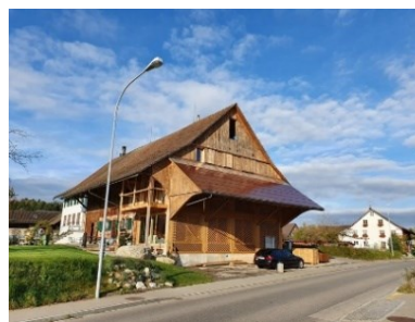
Figure 6. Rural building, Seegräben CH
