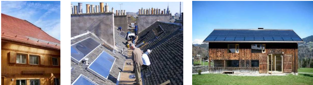
Figure 4: left: colour modules terracotta of PV © Solaragentur Prix Solaire Suisse 2018, Maison rurale Galley, 1730 Ecuwillens/FR; middle: solar thermal units on ten protected blocks of flats in the City of Edinburgh. © HES; right: side view of the House Breuer (Austria) with non-reflecting PV modules with a dark background ©FG Marcello Girardelli
