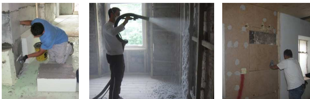
Figure 1: left: installation of internal insulation (Perlite) at Villa Castelli © Eurac; middle: Blowing on the wet cellulose insulation material © HES; right: installation of wood fibre © Eurac
