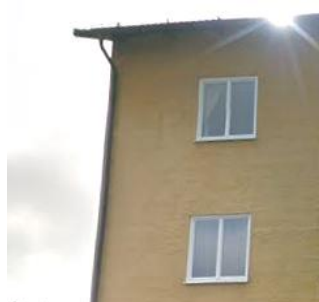
Figure 3. Example of observation in Google Street View of a building with eaves overhang and without brick façade, i.e., a building that is suitable for additional façade insulation.
