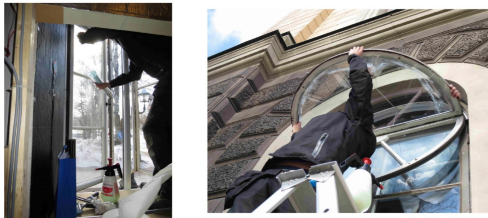
Figure 7. Installation of the low-E window film on surface 3 [33].
