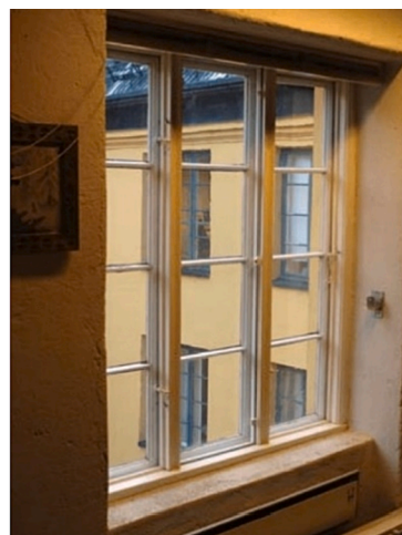
Fig. 3.1. Installation of a secondary glazing improving the window's U-value from 4.6 W/(m 2 K) to 1.6 W/(m 2 K). Photo: Marte Boro [125].
