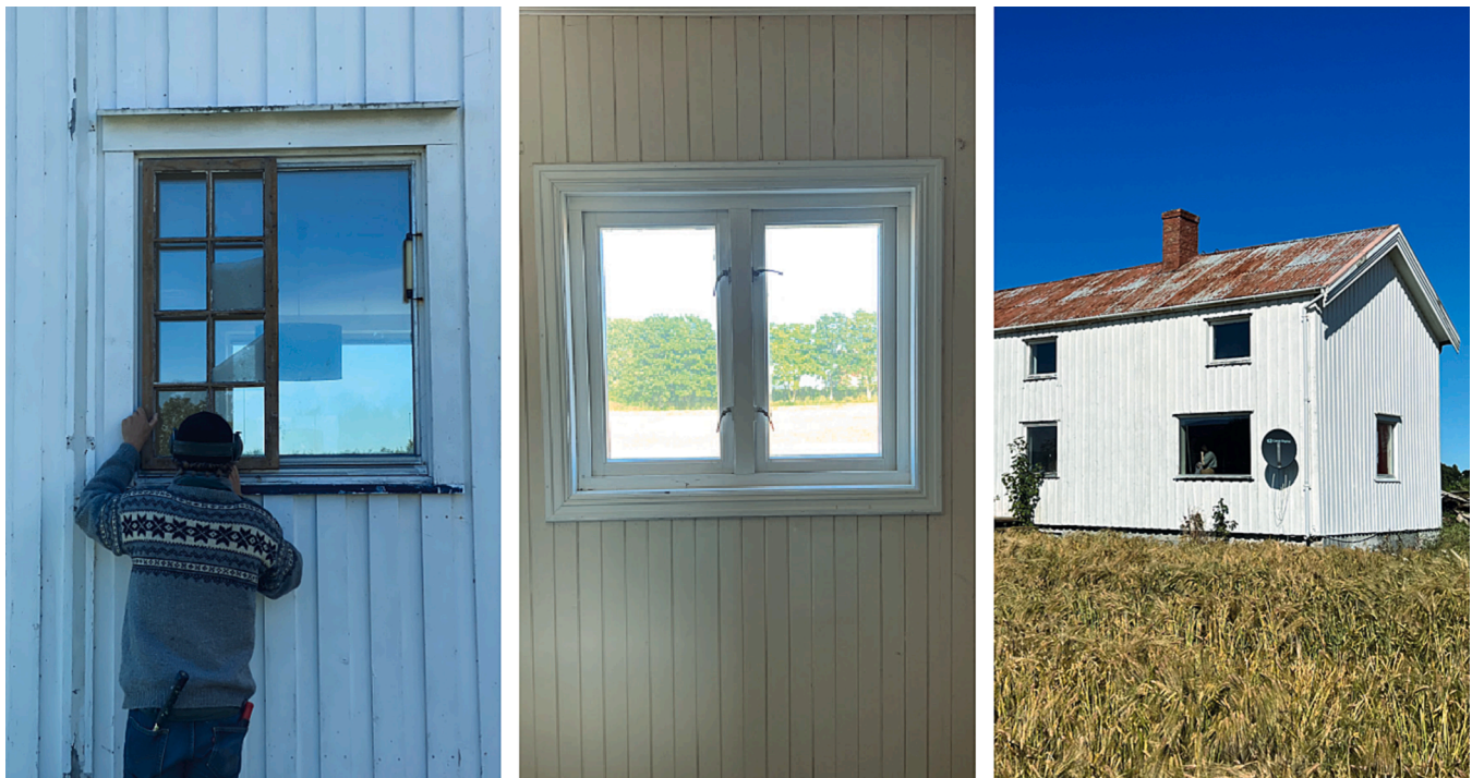
Fig. 6.13. Left: Old slatted window found at the farm held over an awning window of Grande. Middle: two-section casement window of Grande. Right: Awning windows on the southwest and southeast façades of Grande. Photos: [49].
