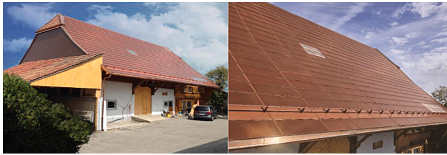
Fig. 5.1. Rural farmhouse in Switzerland from 1859 with terracotta coloured BIPV (right photo). The left photo shows the building before the energy upgrade. Photos from [75].
