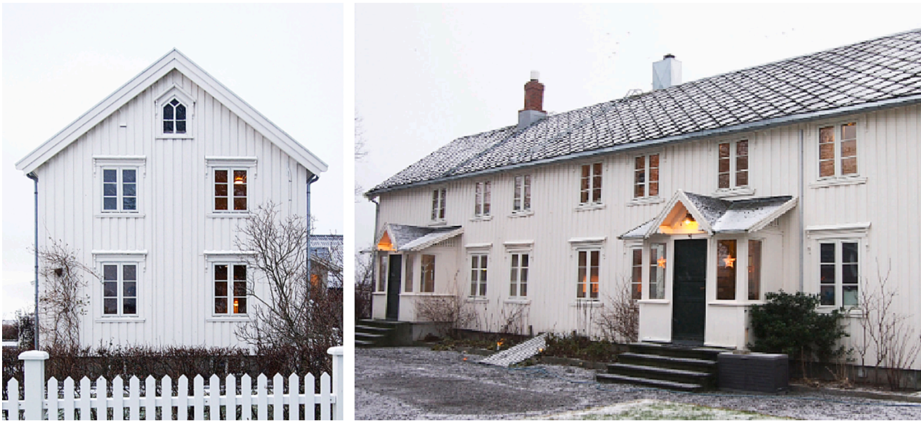
Fig. 6.14. The east (left) and north (right) façade of Viken depicting the current windows [107].
