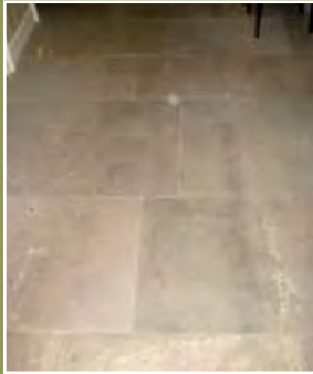
Original flagstone floor.
