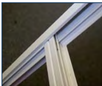
The secondary glazing system installed for the pilot study.
