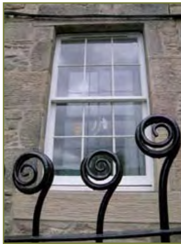
Example of the 'double reflection' caused by some secondary glazing.
