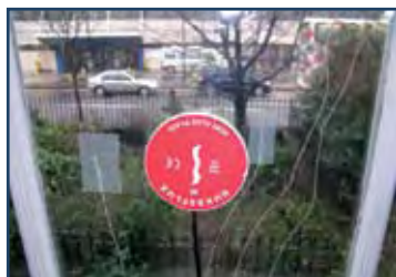
Temperature and heat flow monitoring equipment installed on single glazed window.
