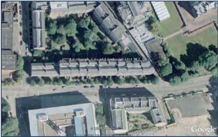
Lister housing Co-operative tenements from above. Image courtesy of Google Earth. Image © 2008 The GeoInformation Group © 2008 Tele Atlas
