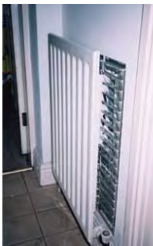
Reflective panel behind radiator
