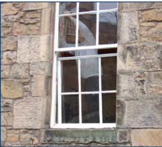
Draughtproofing being installed for the pilot study. Photograph © Changeworks
