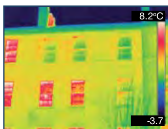
The three top windows have both secondary glazing and internal shutters
