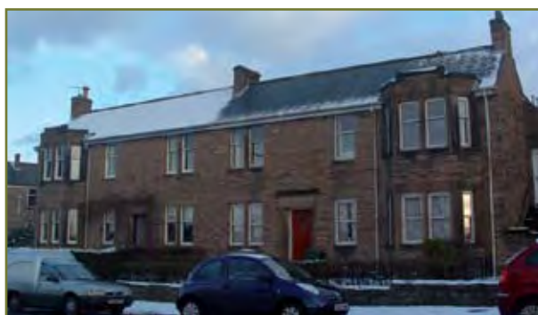
Snow melt caused by heat loss through an uninsulated roof. Photograph © Changeworks
