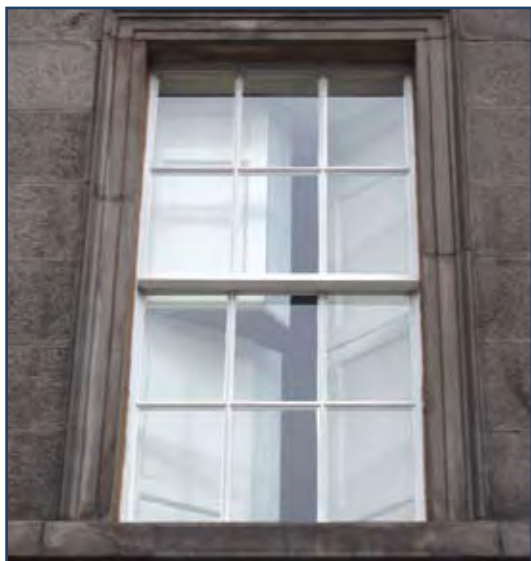
Internal shutters installed for the pilot study.
