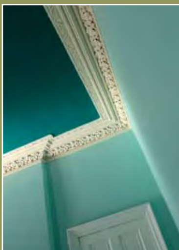
Ceiling cornice in a Georgian tenement
