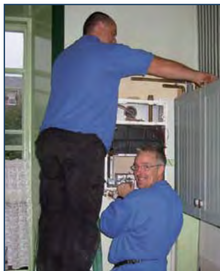
Condensing boiler being installed for the pilot study. Photograph © Lister Housing Co-operative
