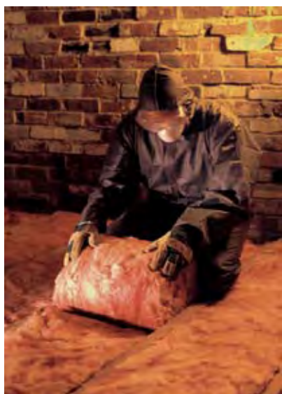
Quilt insulation being installed in a loft. Photograph © Changeworks
