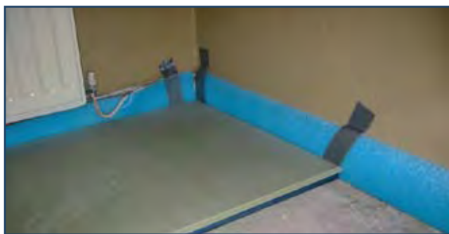
Floor insulation being installed.
