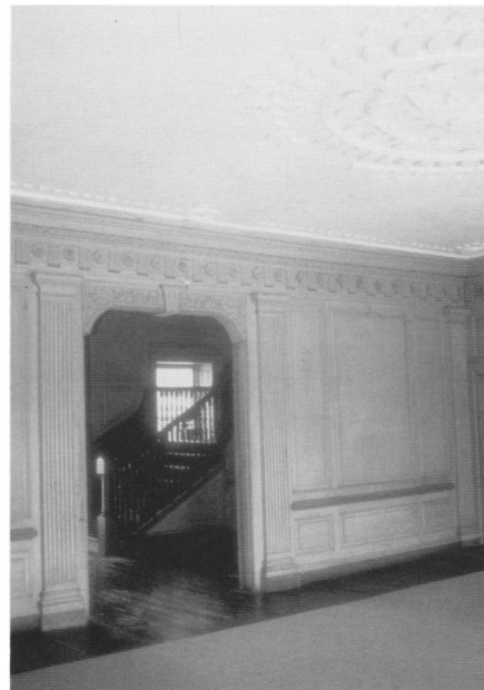
Fig. 3. The Great Hall looking north toward the archway to the stair hall.
