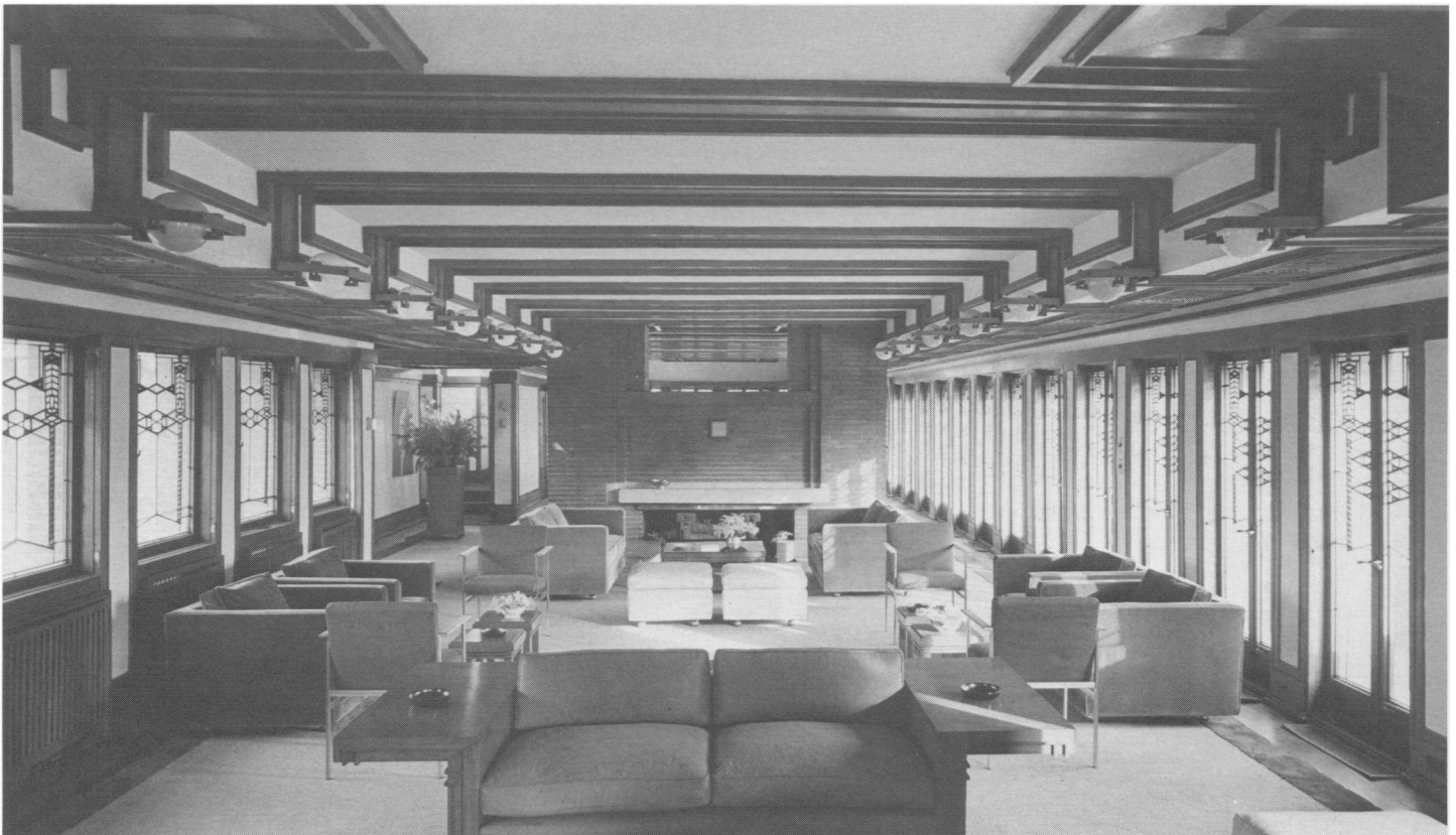
Beneath each window on the left is a fan-coil radiator unit, hidden behind a wooden grille. (Richard Nickel, courtesy of Richard Nickel Committee)
