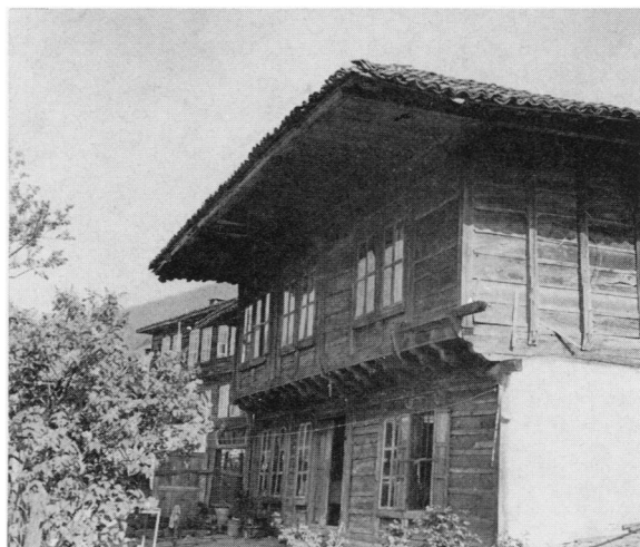
FIG. 1 A typical Bulgarian renaissance house in Zeravna
