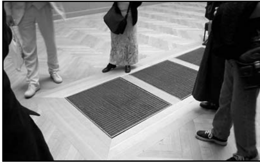
Existing natural ventilation systems in Herzog-Anton-Ulrich, Braunschweig. Above: Air inlet integrated in the floor. Below: Skylights for daylighting and extraction of used air
