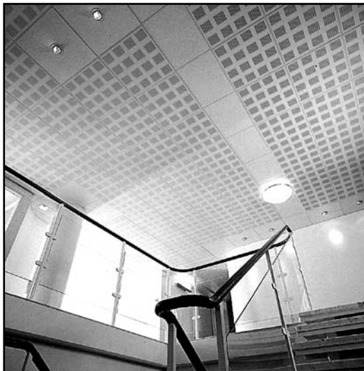
Example of an installation of Gyptone
