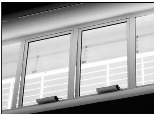
Delphi ventilation - automatic windows
