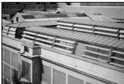
Automatic light control louvres on gallery roof
