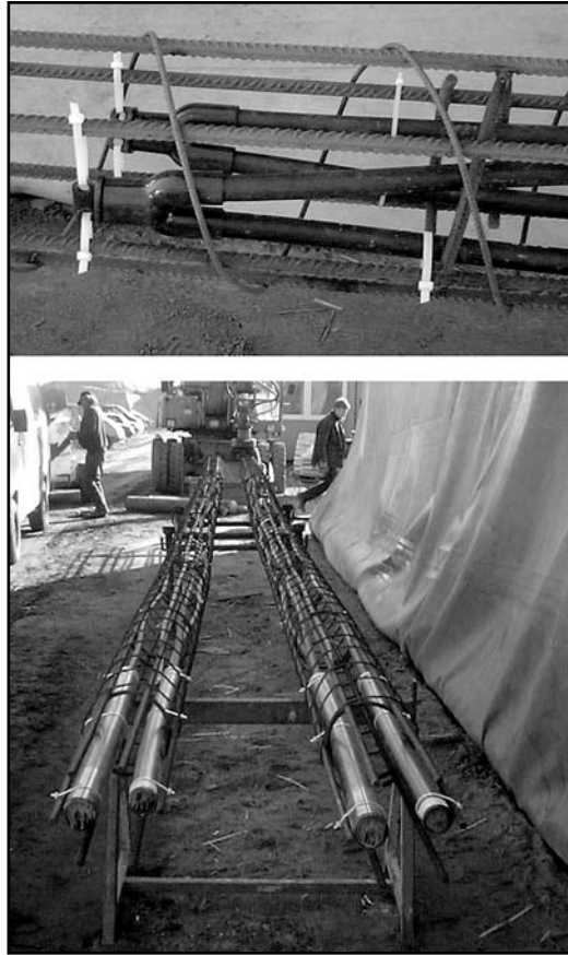
Reinforcement and U-tubes of energy piles
