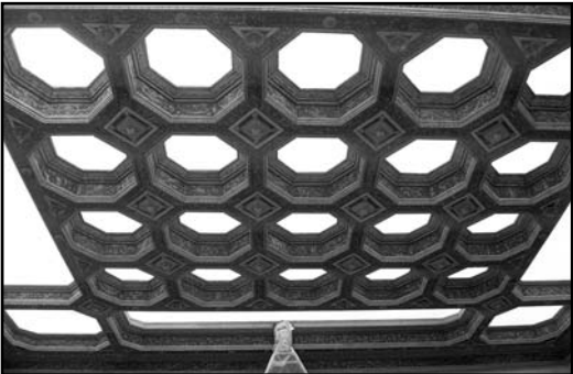
The diffuser panels installed on the old wood ceiling
