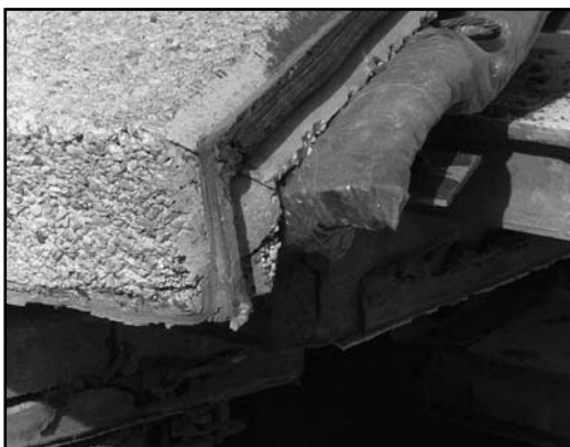
Top: An apartment building from the 1960s being recycled. Middle and bottom: It can be deconstructed - but a closer look shows that the sealants contains large amounts of PCB which makes it difficult and expensive to reuse the components
