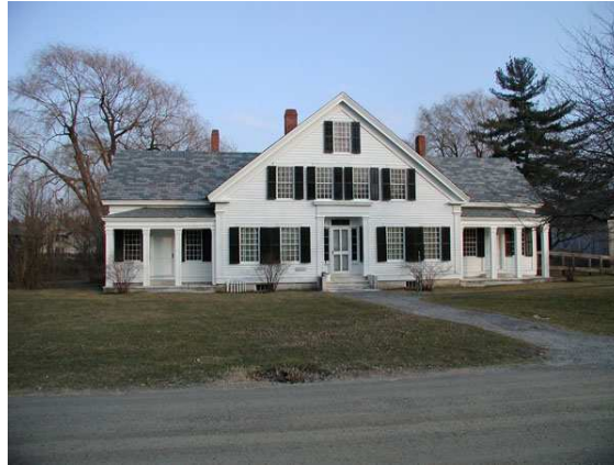
Figure 4. Class 4 Building, Dorset House.
