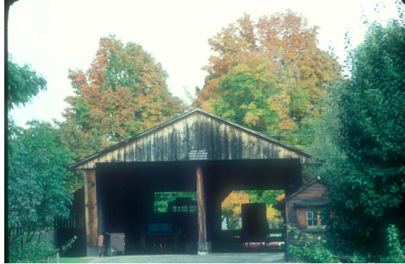
Figure 1. Class 1 Building, Cambridge Covered Bridge.
