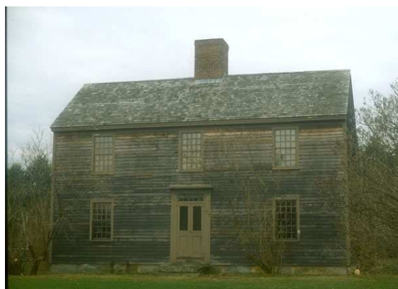
Figure 3. Class 3 Building, Prentis House.
