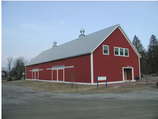
Figure 8. Collections Management Building.
