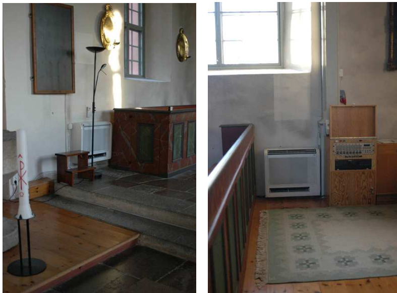
Figure 2. The location of the heat pumps.
