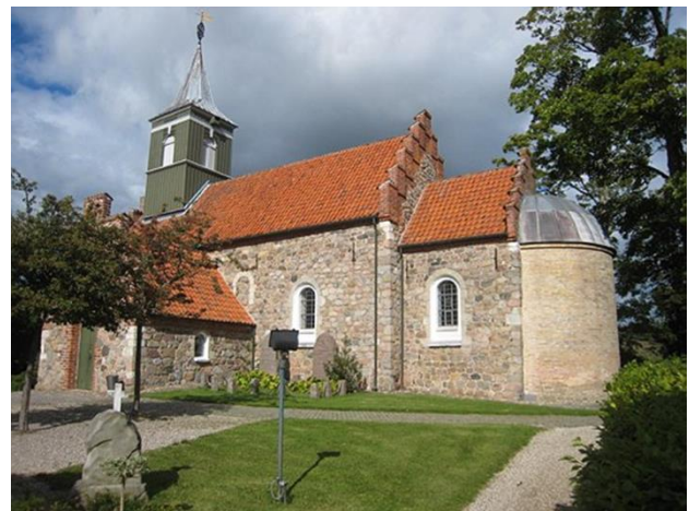
Figure 2 Exterior view of Nødebo Church from the south east. Solar heating of the interior through the small windows is too little to heat up the interior in summer.
