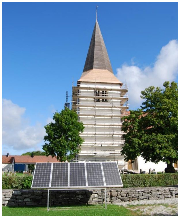
Figure 8 . Exterior view of Hangvar Church from the south. The photovoltaic elements for preheating the inlet air is located outside the churchyard fence.
