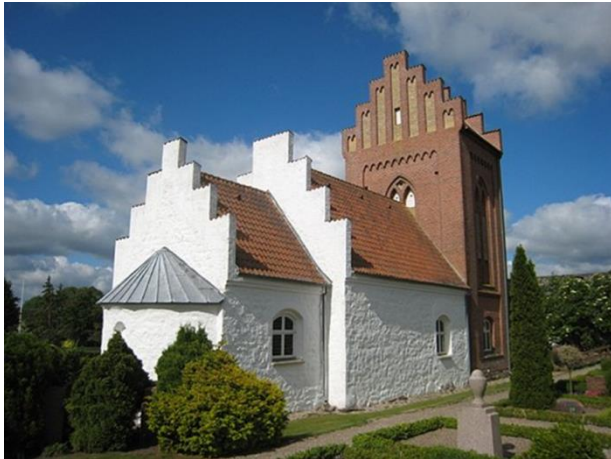
Figure 6 . Exterior view of Tyvelse Church from the northeast. The air supply to the nave and chancel was drawn from the attic to gain heat from the solar radiation to the tiled roof.
