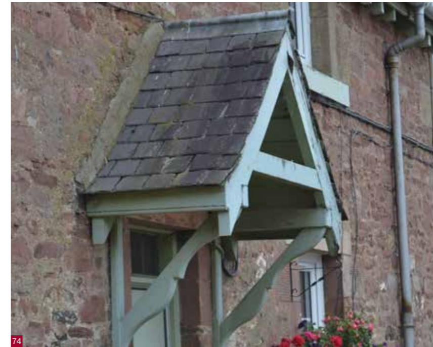
Fig. 74 A decorative porch canopy from the late 19th century.
