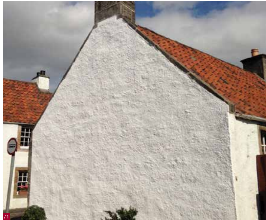
Fig. 71 Limewashing of masonry elevations consolidates the masonry units and the mortar.
