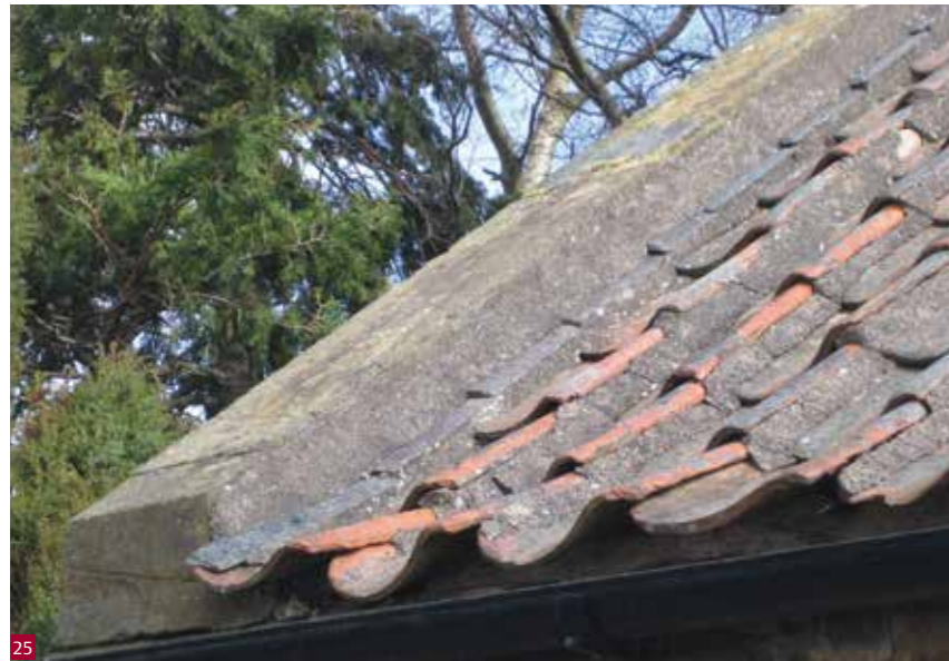
Fig. 25 Mortar torching on pantiles to prevent wind lift.
