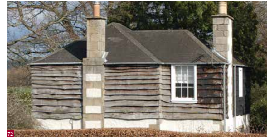
Fig. 72 External timber cladding to a building in the Scottish Borders.
