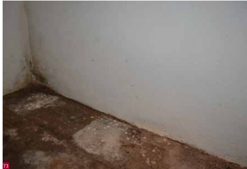
Fig. 73 Lime plaster finish used in a basement.
