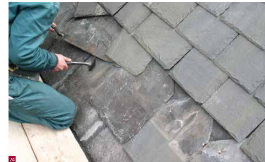
Fig. 24 Fixing slates with additional fastenings to prevent wind lift.
