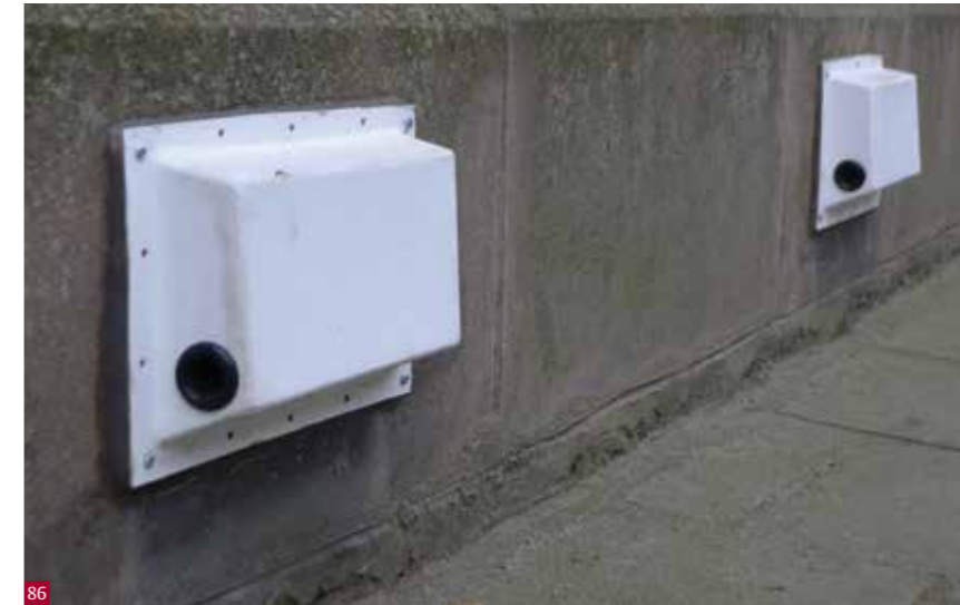
Fig. 86 Temporary barriers can be fitted over openings in flood-risk areas © Paul Hendy.
