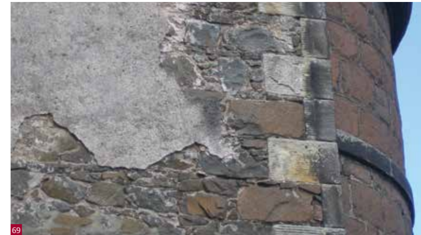
Fig. 69 Traces of original render on the gable end of a late 18th century building in Stirling.
