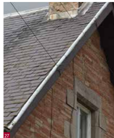
Fig. 26 Edge of slate cut to drive water away from the junction and minimise run off onto the gable.
