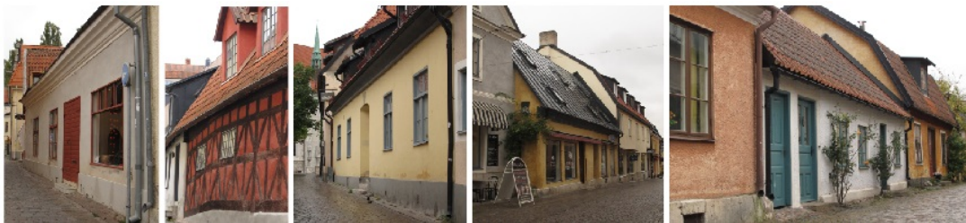
Figure 23: The terraced Category 1c buildings have similar characteristics compared to Category 1a and 1b, but are not necessarily as old.
