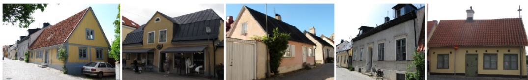
Figure 20: Five typical volumes and exteriors of Category 1b buildings.
