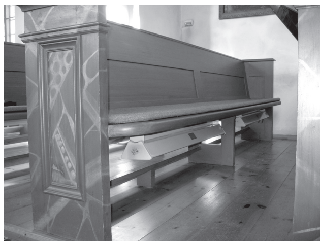
Fig. 3. Three photos showing heat pumps HP1 and HP2 and bench heaters.
