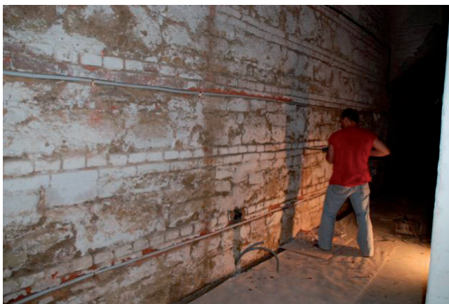
Fig. 8. Simple wall heating in the depot against humidity and for climate stability.
