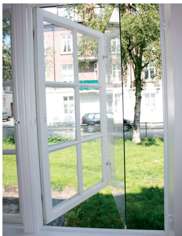
Fig. 4. Energy calculations showed that the energy performance could be improved significantly, for example by mounting double glazing with low-emittive panes. The illustration shows use of Opto-Glas, a Danish frameless system. Photo: Ingun Hopen.
