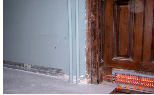
Fig. 7. New convectors under the historic windows.
