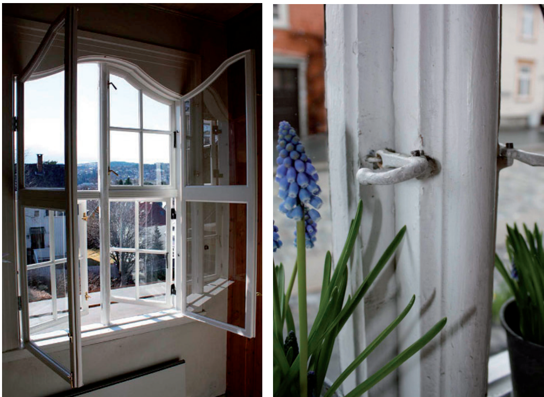
Fig. 3. Original windows are significant architectural elements, often with high-quality materials and excellent detailing. Secondary glazing systems are often part of the original window.
