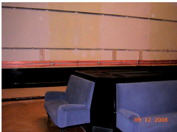
Fig. 23. Wall heating on the cold outer wall.
