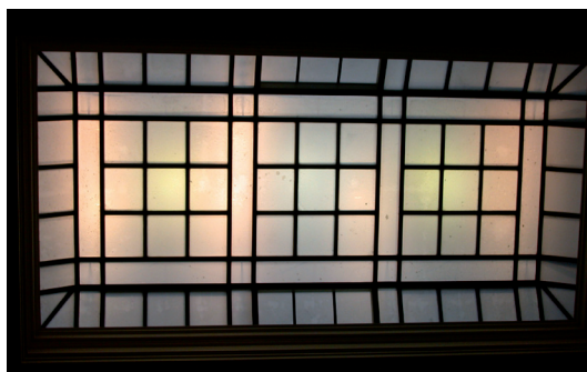
Fig. 4. Skylight roof with a combination of natural and artificial light – Non-uniform light source distribution and light colour. Photo: Anke Schenk.
