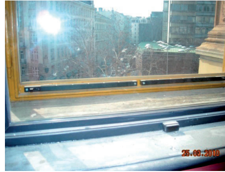
Fig. 3. Summer ventilation system of the shading in the box window.
